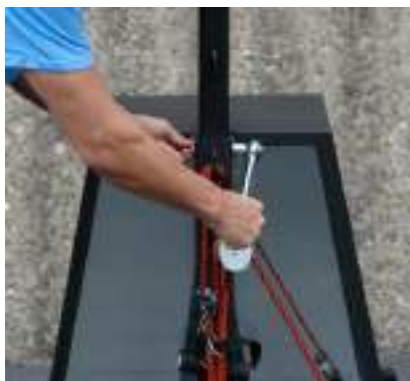
15. Secure the vertical post to the housing using two 3/8" x 3" long bolts.
