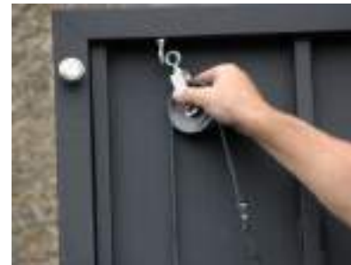
11. Be sure that the rewind cord and rubber tubing are not twisted.
