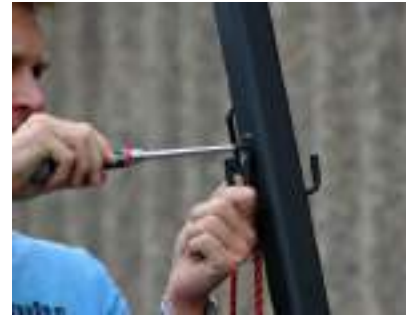
17. Using Philips head screw driver, attach (2) accessory holding hooks to vertical post.
